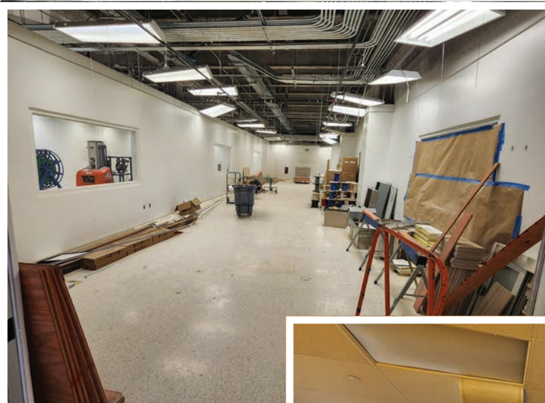
Construction of lab space for labs moving over from Ruby Hospital
